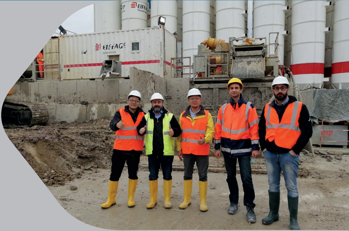
D-wall and works of Grand Paris Express Project
