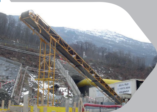
Application in tunneling works
